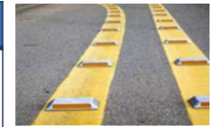
Raised reflective pavement markers (RRPMs)
