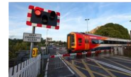
Railway crossing upgrade
