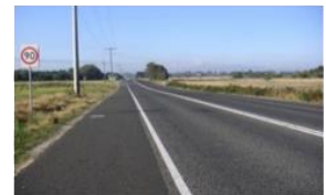
Shoulder widening and/or sealing
