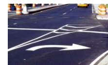
Painted turn lanes
