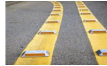
Raised reflective pavement markers
