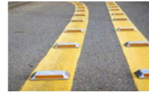
Raised reflective pavement markers (RRPMs)
