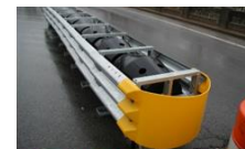
Crash cushion/impact attenuator
