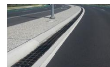
Pavement drainage improvements
