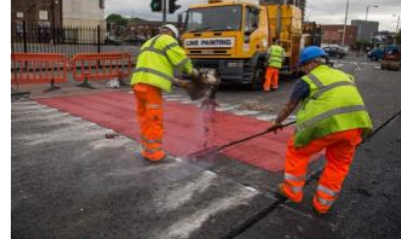
Skid resistance improvements
