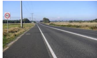
Shoulder widening and/or sealing
