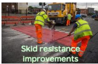
Skid resistance improvements
