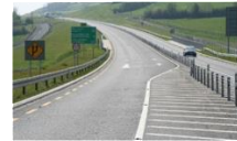
Additional lanes for overtaking
