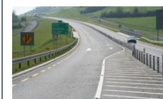
Additional lanes for overtaking
